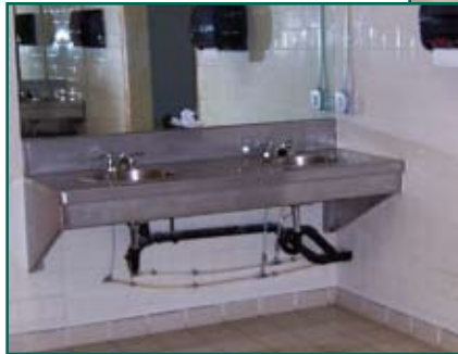
stainless steel sinks and counters located in the NDTC dormitory.
